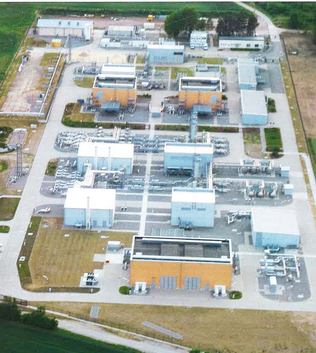
Bird's-eye view of Storengy's Peckensen natural gas storage site. The company is the number 1 storage operator in Europe and number 4 in the world.
