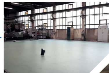
Subsequently, the floor was also renewed.
