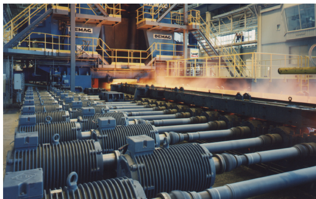
Figure 1: Wide hot strip mill train, ARC 315
